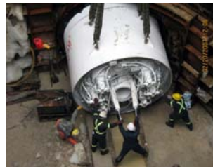
Tunnel Boring Machine
